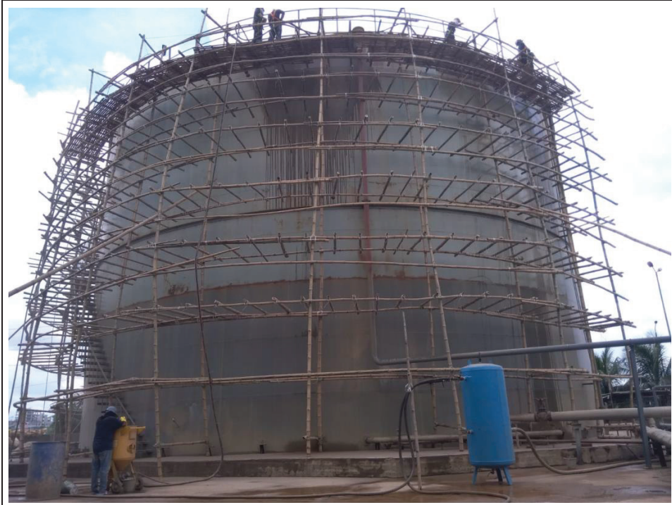
1. Erected bamboo scaffolding and blasting tank HFO Tank No. 1
