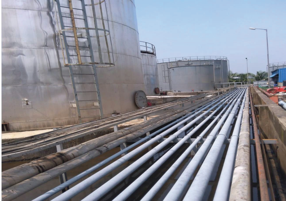
3. Blasted and applied Zinga on the associated pipes
