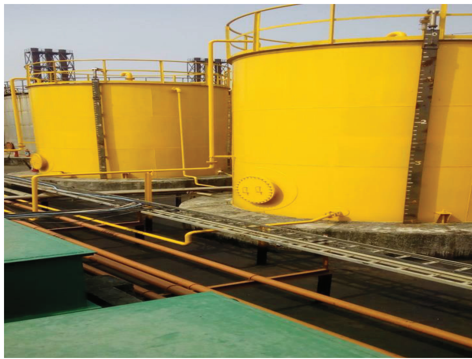
11. Top PU coating 50-60 micron completed.
