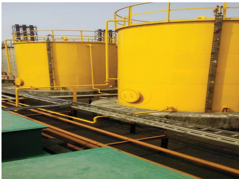
16. Top PU coating 50-60 micron completed.
