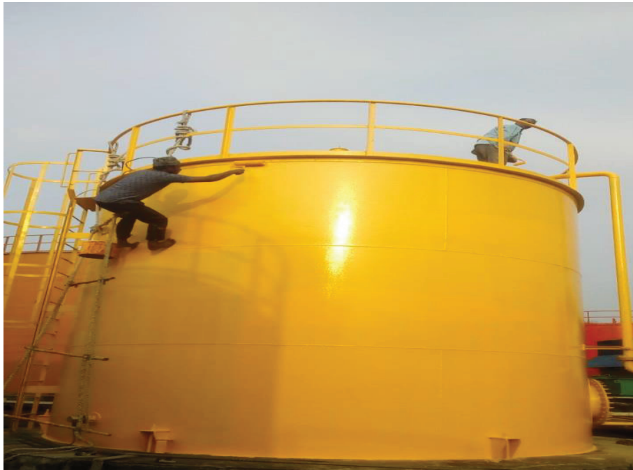
14. Top PU coating 50-60 micron completed.
