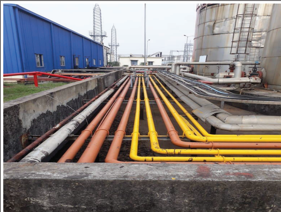
15. Top PU coating 50-60 micron completed.
