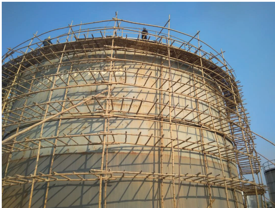
2. Erected bamboo scaffolding and blasting tank HFO Tank No. 2
