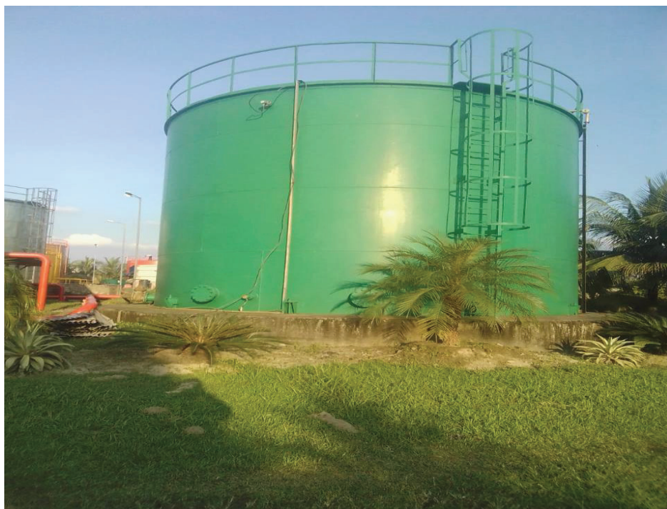
13. Top PU coating 50-60 micron completed.
