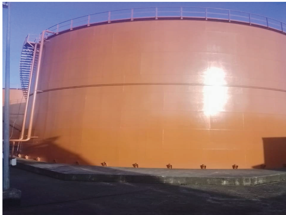
12. Top PU coating 50-60 micron completed.
